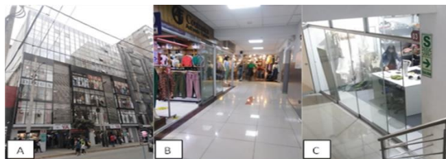
Figure 11. Multi-purpose building Ya, warehouses, and internal offices.
