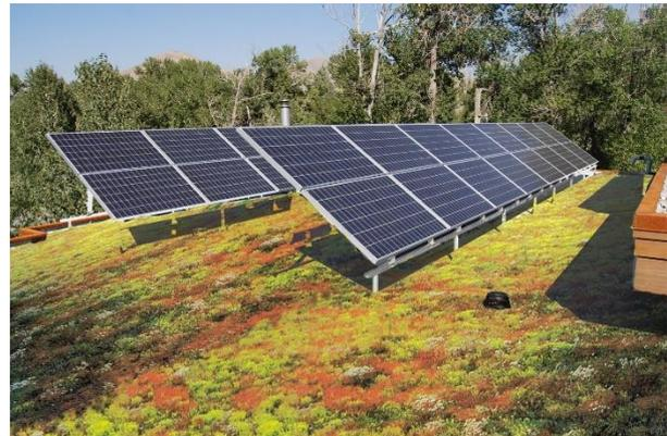
Figure 1. Integration of PV panels on the green roof.
